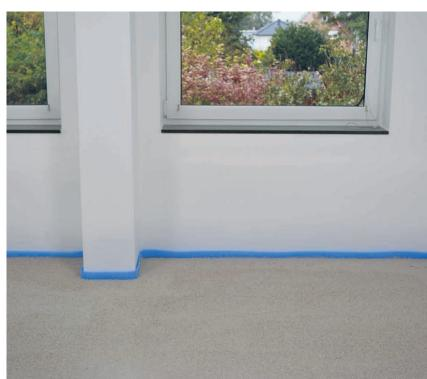
After 12 hours drying time, the area can be walked on, and after 3 - 4 days, it can be laid. Observe: CompactFloor THERM CE is not a finished usable layer on which floor coverings can be directly laid.
