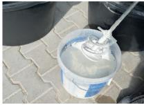
Stir water (3.75 litres) and CE binder (1 sack) into a bucket with an agitator at medium speed.
