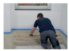
Strip the surface, retaining the height profile.
