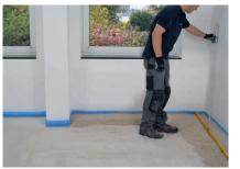
Form dams based on the metre level in the height profile. Layer thickness at least 30 mm to max. 500 mm.
