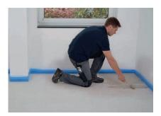
Lay out the edge insulation strips, carefully clean the subsurface and prime for sufficient adhesion with the deep primer.
