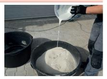
Add the entire contents of the granulate sack into a mortar bucket and add the pre-mixed CE binder.
